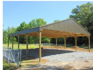
OPEN, POLE BARN
